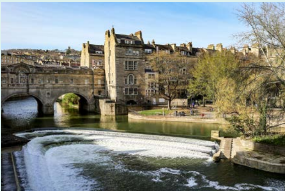
Pulteney Bridge and Weir, Bath
